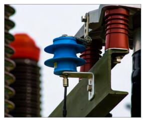
Permanent installed UHF Termination Sensor
